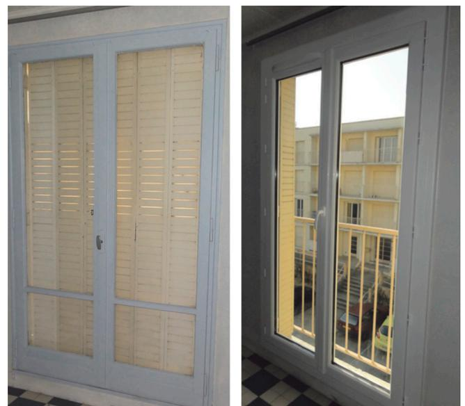
Figure 2. Example of mitigation solution, on the left single-glazed window without trickle vent, on the right double-glazed window with an acoustic trickle vent.
