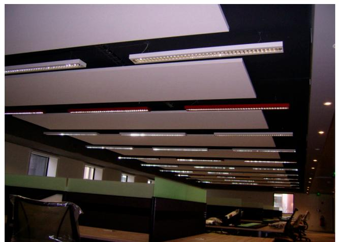
Figure 4. High acoustic performance horizontal free hanging units based on glass wool.
